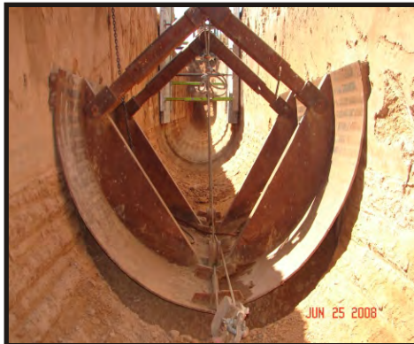
Dig the trench.
