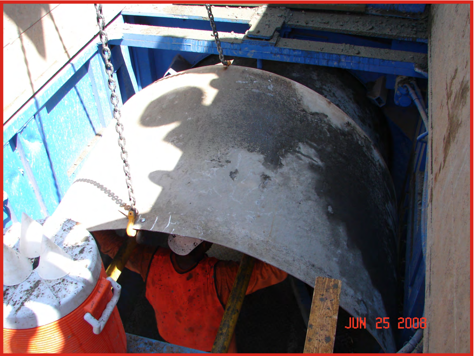
AN ALUMINUM FORM BEING PLACED AND SECURED.
