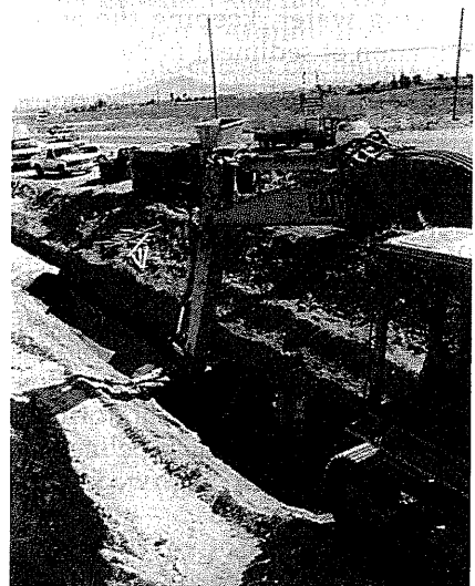
The day after the pour, the supports are collapsed and removed and forms are pulled from the pipe by the excavator. The forms, which are connected to each other when installed, come out upside down after being released from the concrete. Note how the trench conforms precisely to the size and shape of the bucket.
