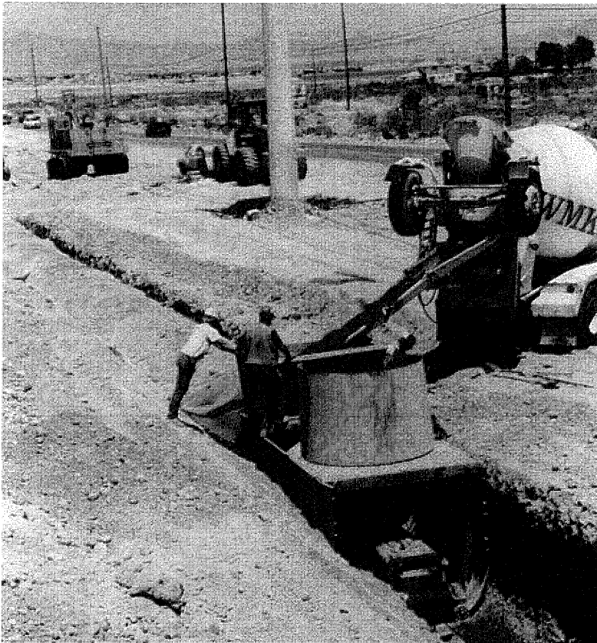
Cast-in-place boat slipforms the concrete pipe. Forms are inserted manually from above.
